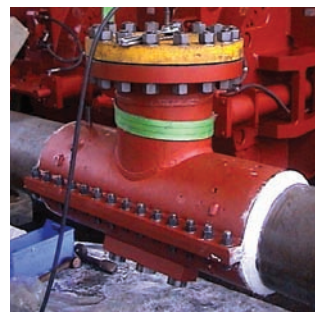
A 12" Grouted Tee fully installed
