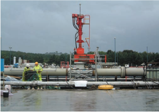
Hot tap field installation
