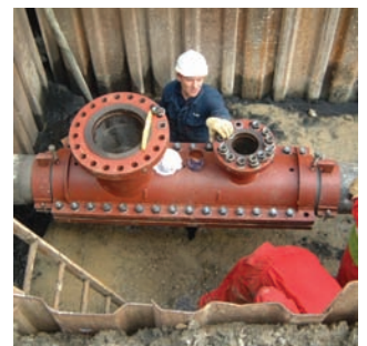
Installation of double branch Grouted tee
